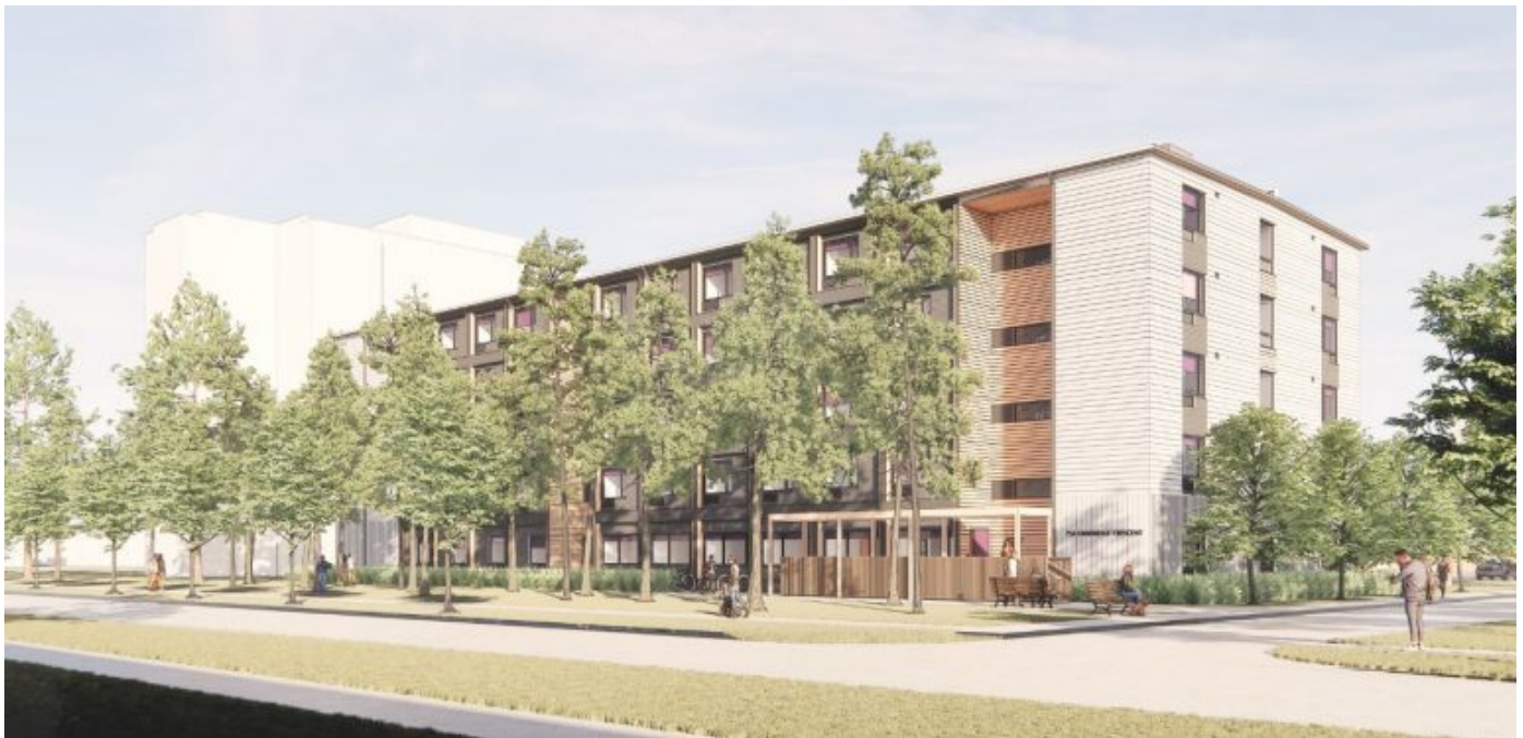
Image Three: Preliminary artist’s rendering of the modular building – Looking East on Tandridge Crescent. Final design subject to approval.
