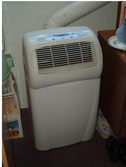
Portable air conditioners require additional cooling capacity to effectively cool the same space because the entire unit is located inside the space being cooled, not
